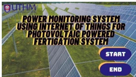
Figure 22.3 Example of the solar monitoring system in application
